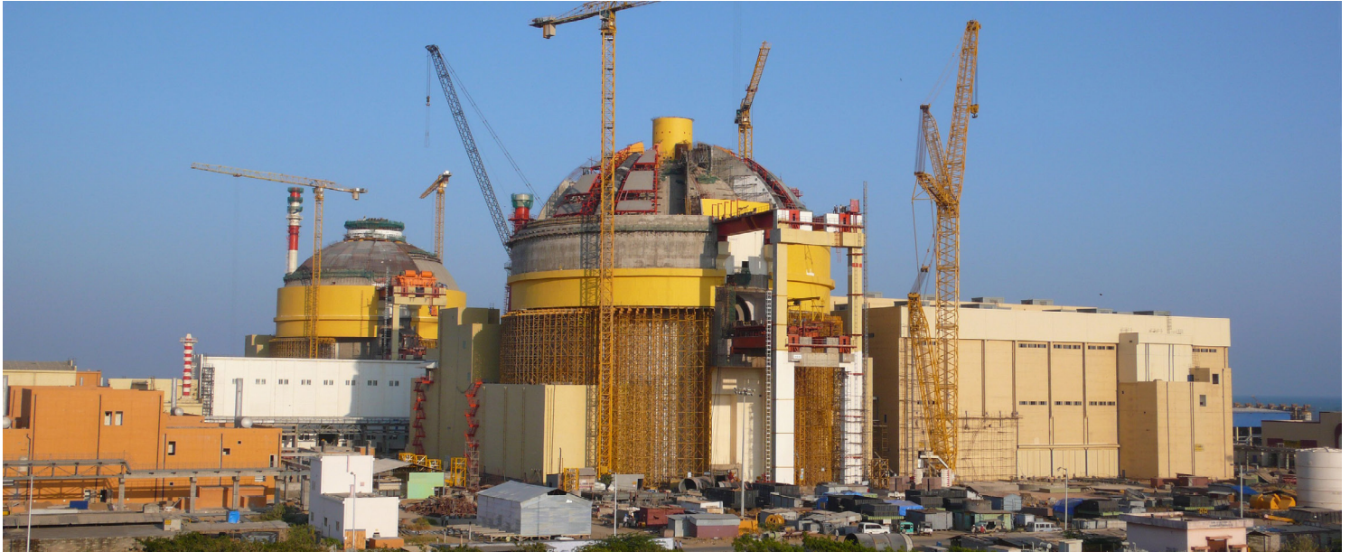
Nuclear power plants under construction. Photo: Petr Pavlicek / IAEA imagebank@Flickr
